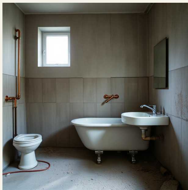
BATHROOM STRIPPED BACK DURING WORKS - CONDITION DRIVES COST - ILLUSTRATIVE
