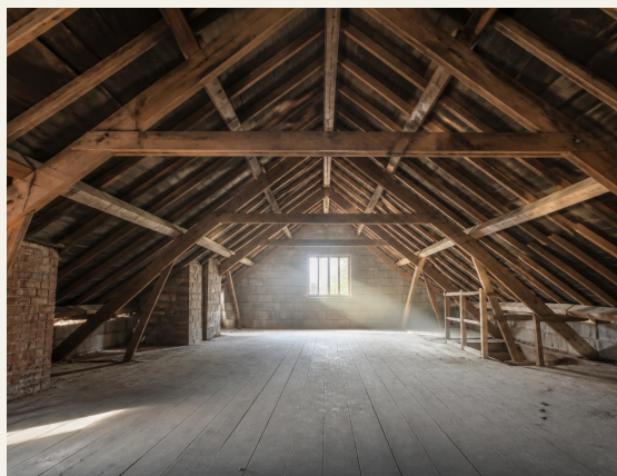
UNUSED ROOF SPACE PRIOR TO CONVERSION - ILLUSTRATIVE
