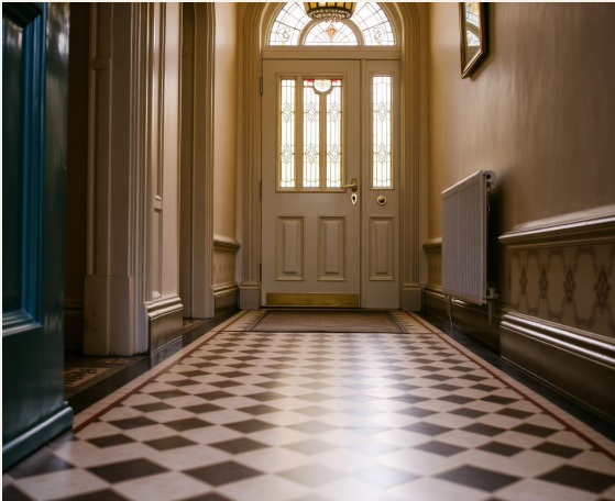
ORIGINAL TILED ENTRANCE HALL IN A PROPERTY UNDER INDEPENDENT SURVEY - ILLUSTRATIVE
