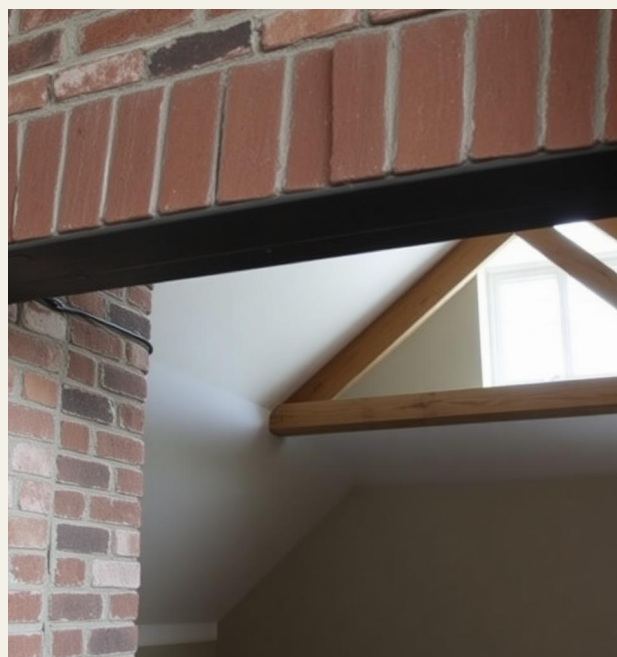
STEEL BEAM OVER A NEW STRUCTURAL OPENING - CONDITION INFORMS VALUATION - ILLUSTRATIVE
